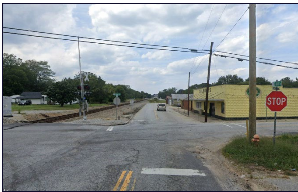
Site 1 – Existing Conditions
