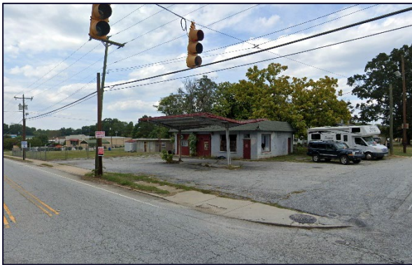
Site 2 – Existing Conditions
